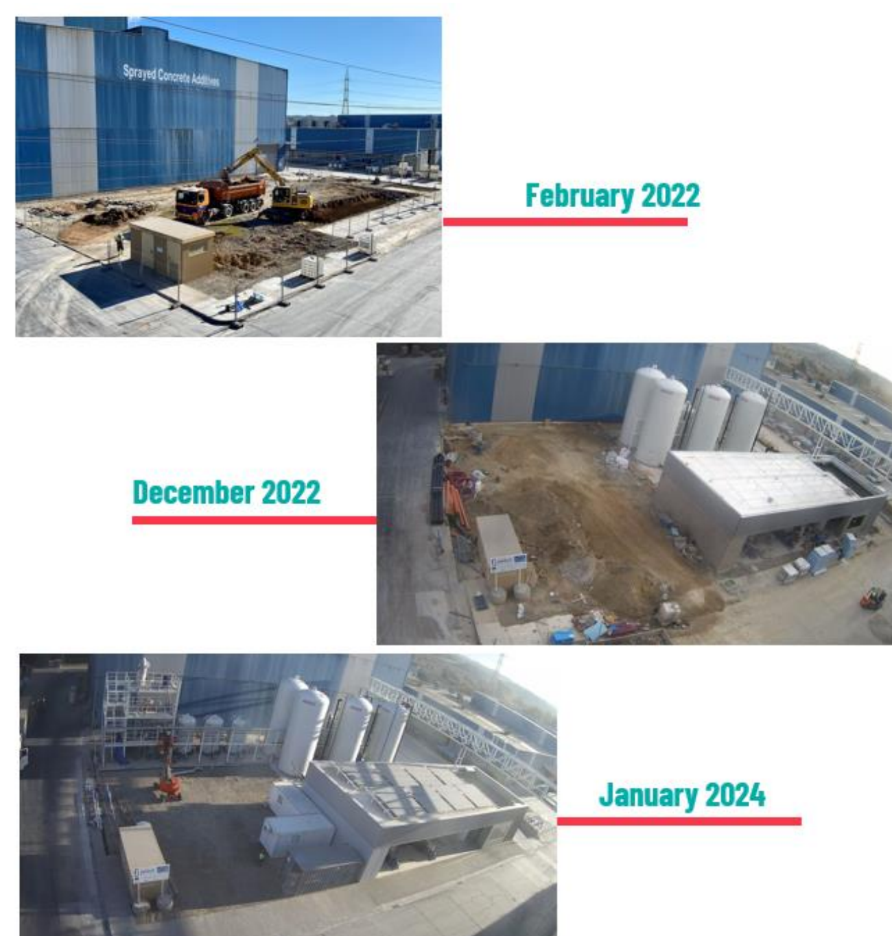
Figure 2. Construction process of the pre-industrial pilot at IQE
